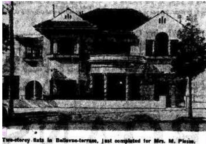
Bonner produced these now-demolished Bellevue Terrace, West Perth flats while with Bohringer, Taylor & Johnson ( The West Australian , 23 June 1928, p.4).
