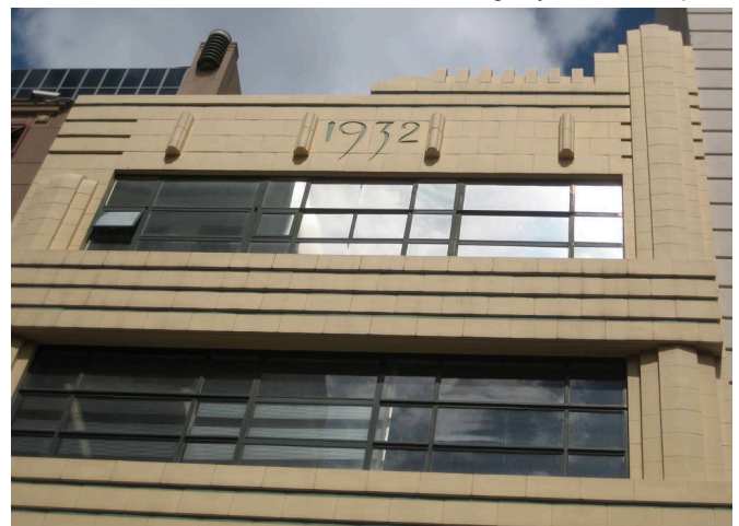
Shows detailing of spandrel panels & parapet 2007, by David Thompson
