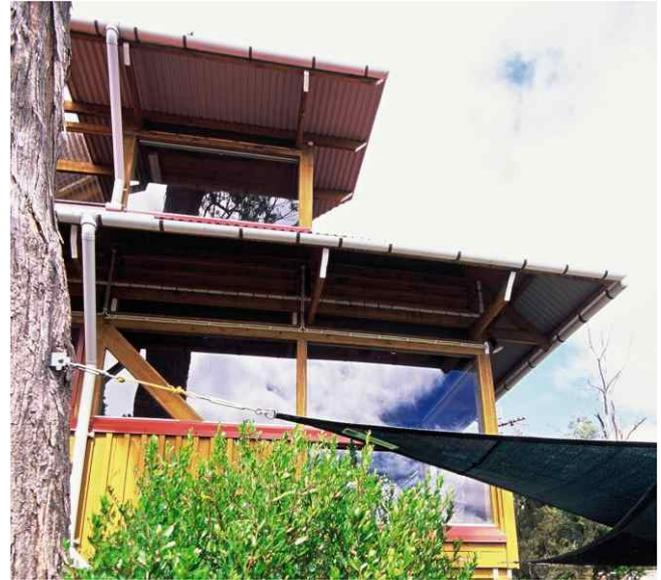
Characteristic timber framed post and beam construction
