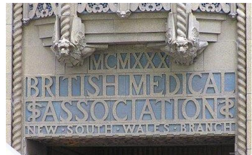
Façade detail showing faience terracotta detailing. (Source: S Watters, NSW Heritage Office)
